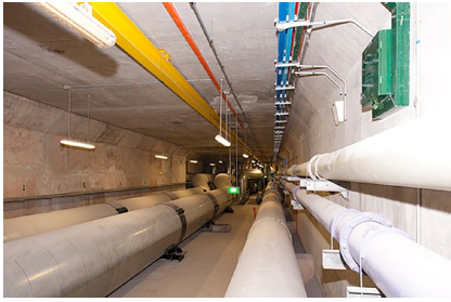
Fig. 04: Common Service Tunnel (CST) [Source: © ctrlshift.gov.sg 17 ]
