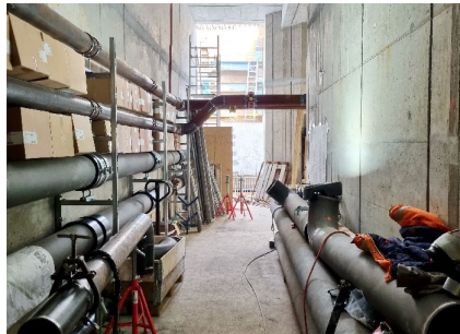
Fig. 03: Inner-city construction, trenchless loose equipment via installation openings [Source: © GIBA mbH]
